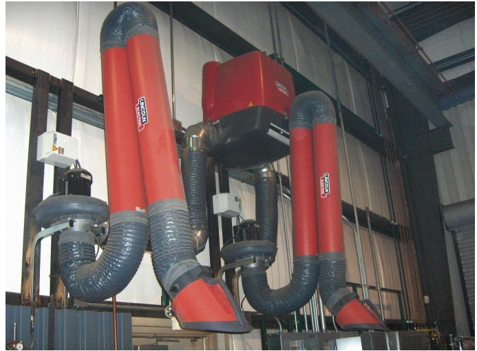
Statiflex® 200-M Dual Arm installation.
